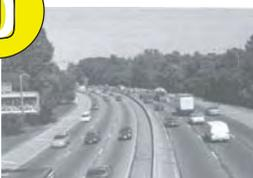
**LOS D** – Represents traffic operations approaching unstable flow with high passing demand and passing capacity near zero, characterized by drivers being severely restricted in maneuverability.
