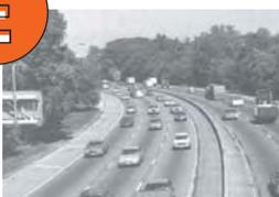
**LOS E** – Represents unstable flow near capacity. LOS E often quickly changes to LOS F because of disturbances (road conditions, accidents, etc.) in traffic flow.
